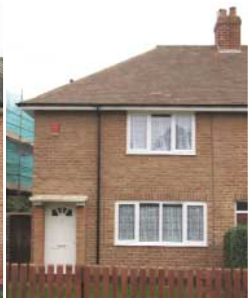
A HOUSE AFTER REPAIR
