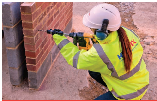
DryFix tie being power-driven into pilot hole
